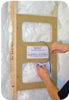
PlaceSaver™ installed during pre-wire phase
